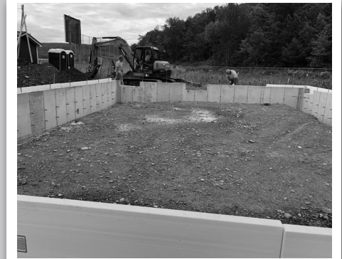
Construction of CV Middle School/High School outdoor classroom
